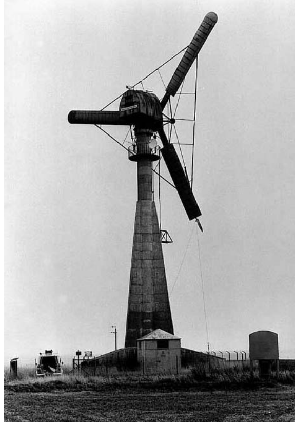
Figure 12. Emergency rotor tip brakes for the Gedser stall controlled wind turbine. Source: Danish Wind Turbine Manufacturers Association.
