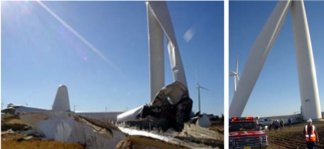
Figure 14. Tower collapse of a wind turbine. Wasco, Oregon, August 27, 2007.
