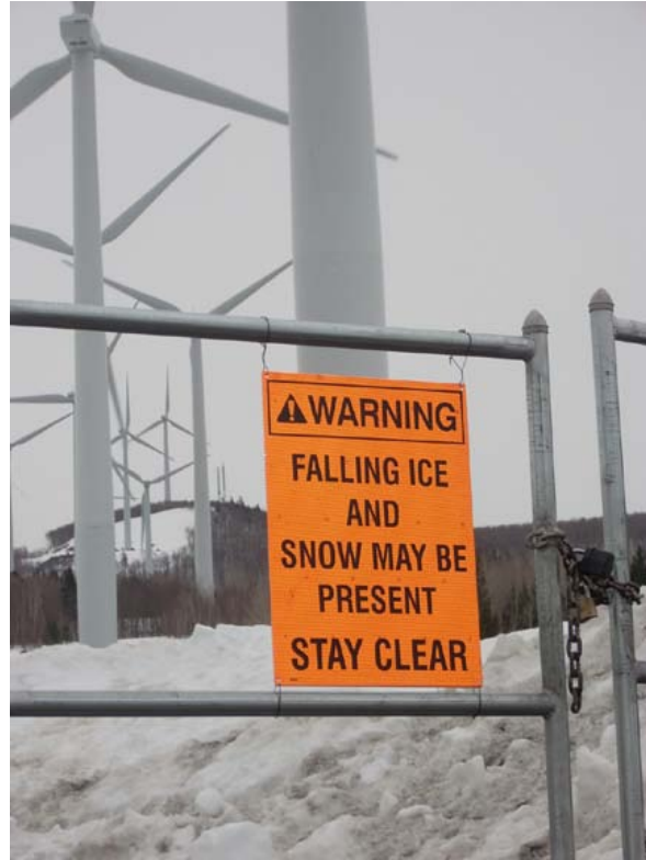
Figure 29. Judicious warning about ice shedding and limited access at a wind turbine site, USA.
