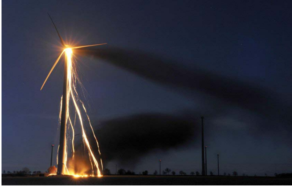
Figure 5. Wind turbine with ignited leaking lubrication oil near Uelzen, Lower Saxony, Germany, December 2, 2009. Source: DPA.
